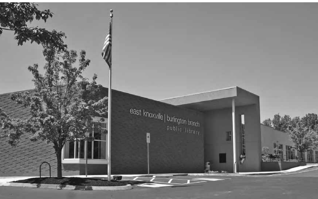
RENOVATION East Knoxville-Burlington Branch Library
