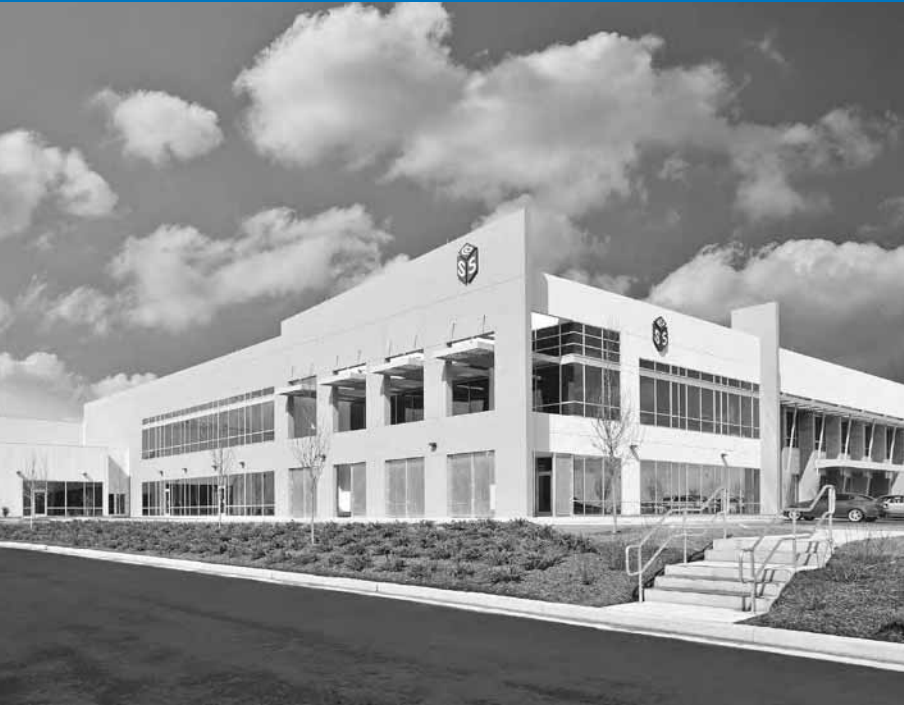
COMMERCIAL/INDUSTRIAL/OFFICE Sysco Food Services of Knoxville
