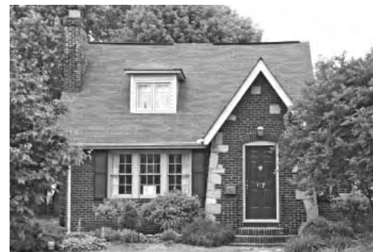
Changes to the zoning in the North City Sector could protect historic homes, such as this one in Adair Gardens.
