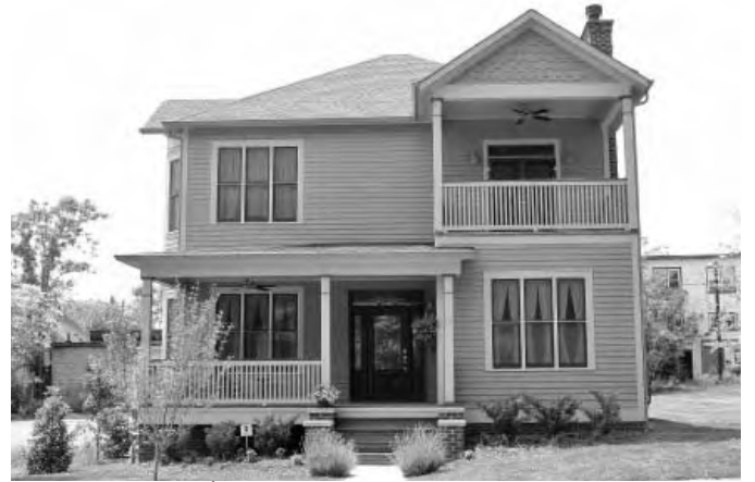
RESIDENTIAL Neff Residence 811 Gratz Street
