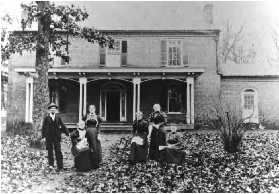
Post Civil War-era photograph of the Kennedy-Baker-Walker-Sherrill House at 9320 Kingston Pike
