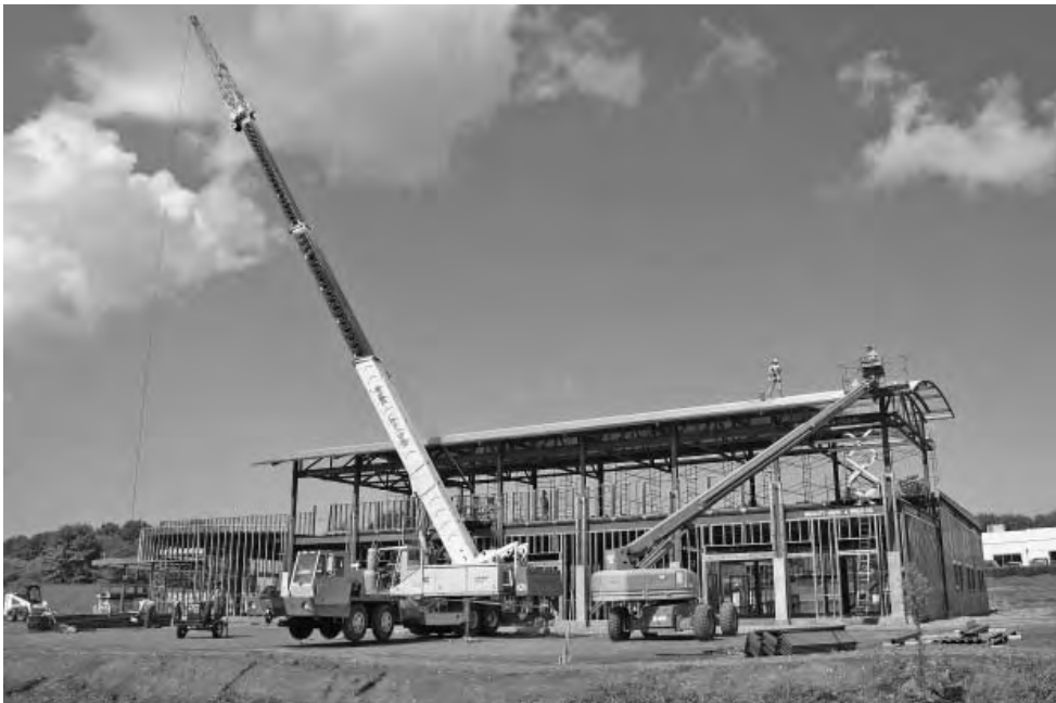
New building construction in the Technology Corridor
