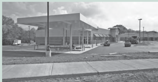
Five Points Village Plaza construction
