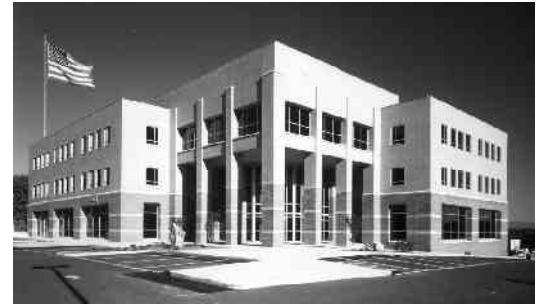
Office: the Summit Building off of North Cedar Bluff Road built by Horne Properties and owned by Grace Commercial Properties
