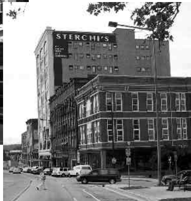
Restoration: the Mill Agent, developed by David and Tracy Dewhirst, and Sterchi Lofts, developed by Leigh Burch, both on Gay Street
