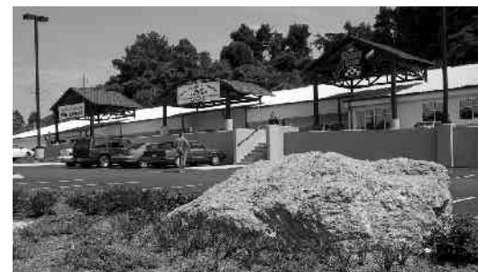
Renovation: South Trader's Landing on Chapman Highway by Chris Gettelfinger
