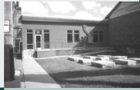
Renovation: Heuristic Workshop at 203 W. Jackson Avenue. Once a train shed, this Old City warehouse is now a modern woodworking shop. The owners are Eric Ohlgren and Carl Keaney.
