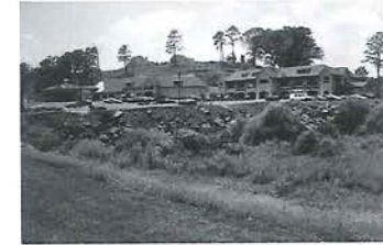
COMMERCIAL Gettysvue Commercial Center 8901 Linksvue Drive Developer: Partners and Associates
