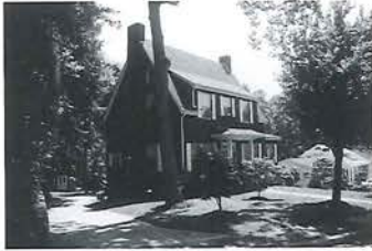
RENOVATION/RESTORATION Thompson-Bridges House 136 Morningside Drive Developer: Angela Bridges
