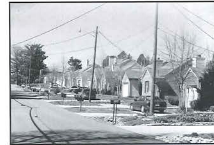
Single family housing in the North City Sector
