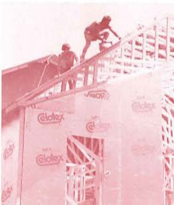
The intensity and type of land use is controlled through the development review process.
