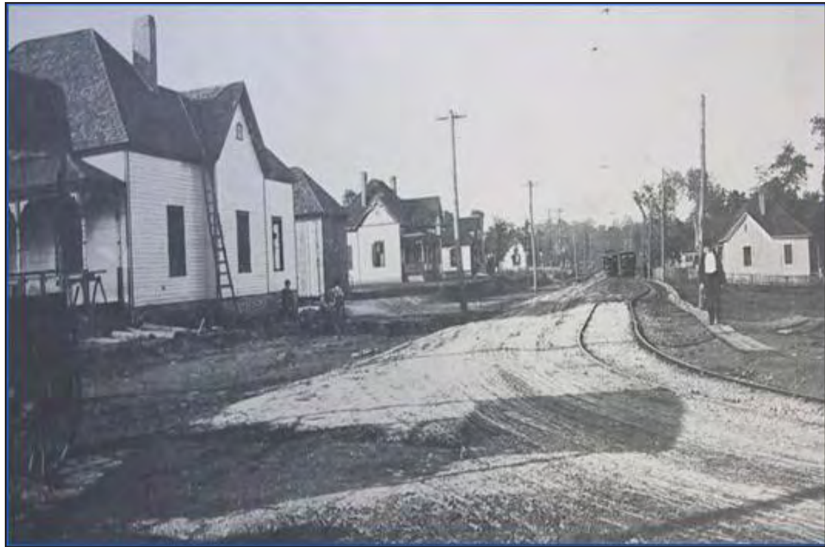
Although the streets have been paved and the board sidewalks replaced, Oakwood's early 20th century housing is still largely intact.
