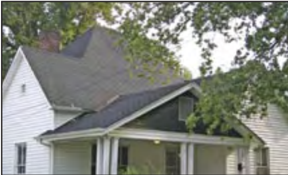
Roof shapes were typically complex. In this case, a Craftsman-style porch joins a hipped-shaped roof.
