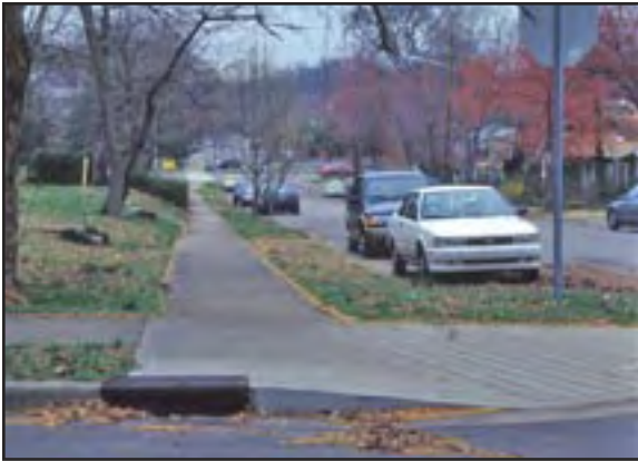
Bulb-outs – A Traffic Calming Device: Corner bulb-outs (shown above in the photo and below in the illustration) function as extensions of street corners for pedestrians and increase protection for vehicles parked on the street.
