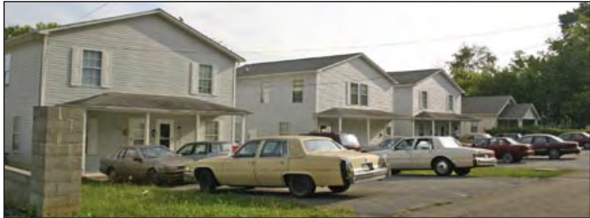
Parking covers the front yards of this infill housing example. If the parking had been off the alley, lawn space and sidewalks would have been possible, matching the historic pattern in most of Lincoln Park.
