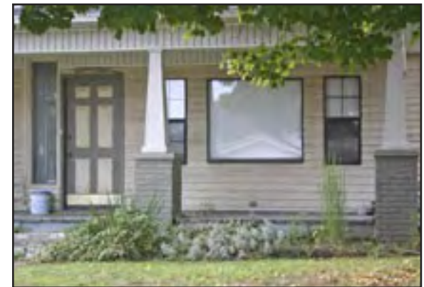
An example where the original style of the windows and doors have been lost
