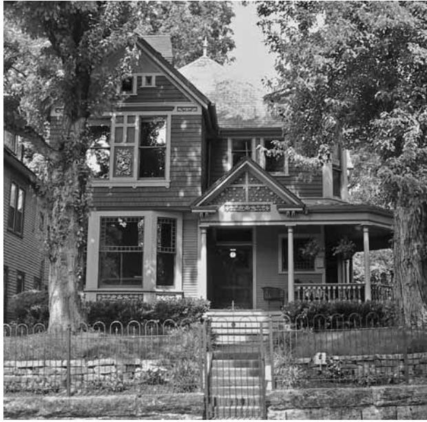
Renovated house in Fourth and Gill
