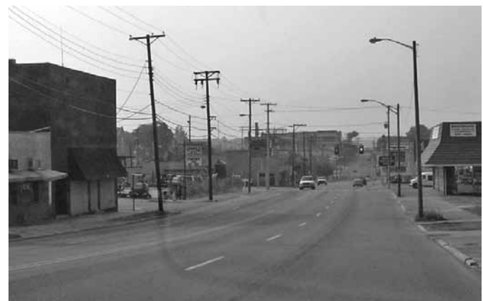
Central Street looking south
