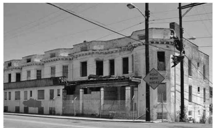
The Mimvilla Flats are going to be renovated and turned into permanent housing by the Volunteer Ministry Center.
