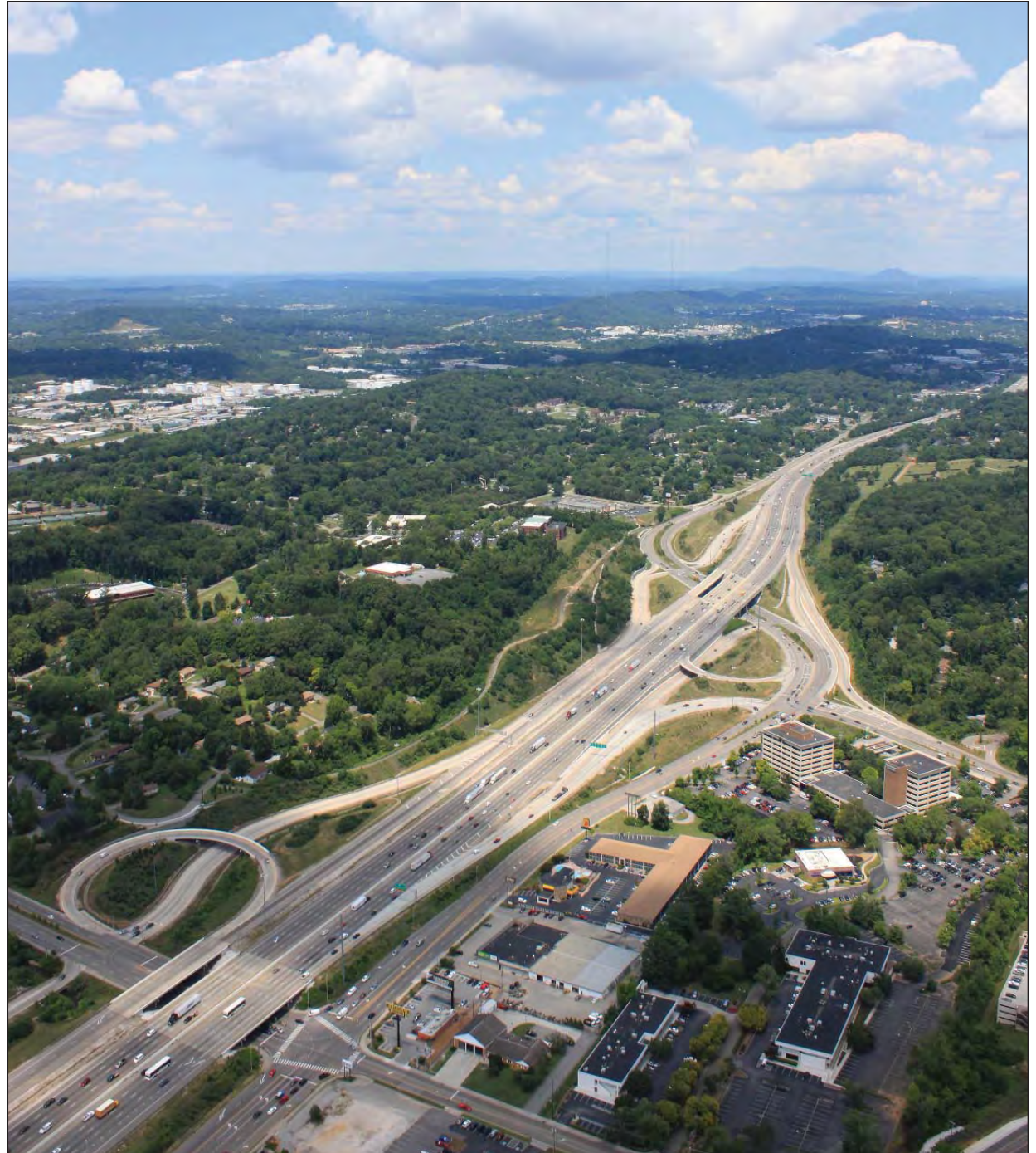
The I-40 Interchange for Papermill and Weisgarber Roads
