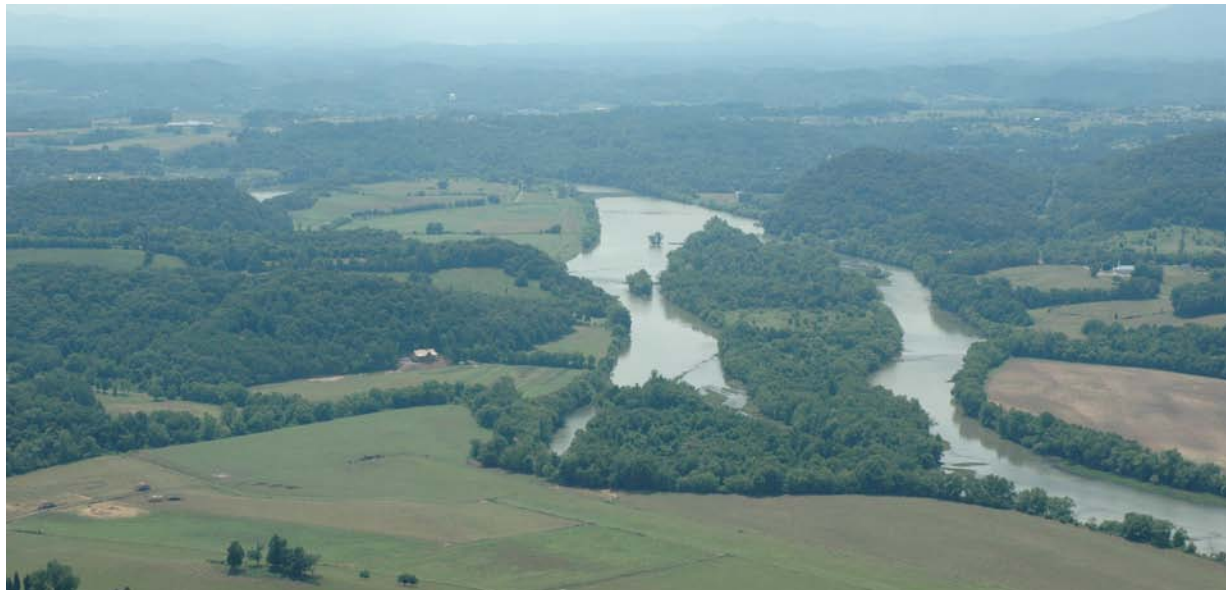
Left: Building a pedestrian bridge across the French Broad River at Seven Islands will provide a tremendous recreation asset to South Knox Countians.
