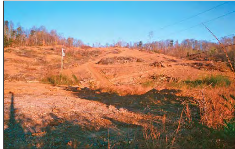
An example of grading where almost all trees were removed
