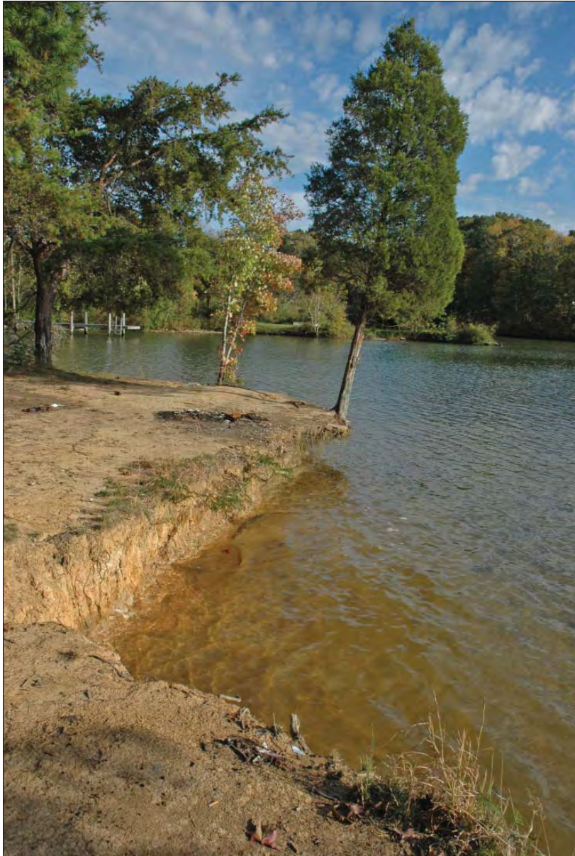
Shoreline erosion increases when trees are lost, like this part of Melton Hill Lake.
