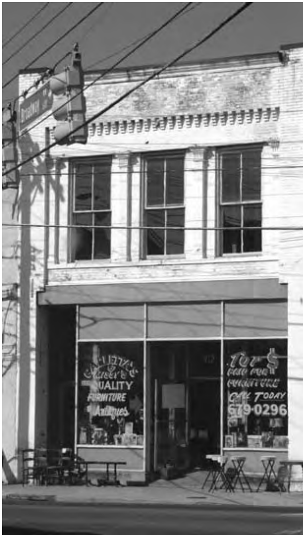
The original features of the ground floor were removed.
