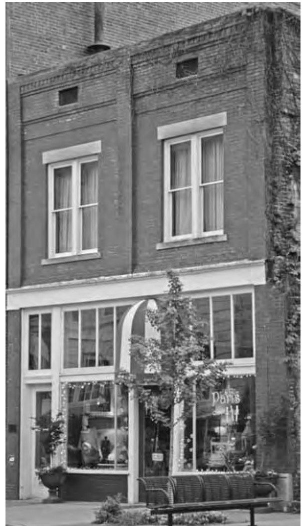
An example of an appropriate rehabilitation.
