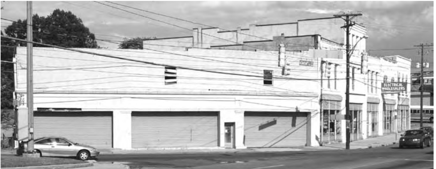
This building at the Broadway-Central intersection is a candidate for facade restoration.
