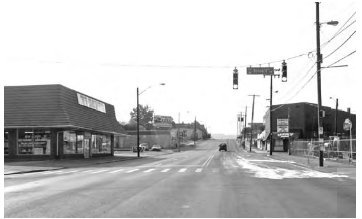
Central Street, south of Baxter Avenue, is an example where the number of lanes is not justified, given the lack of traffic, following I-275 construction.
