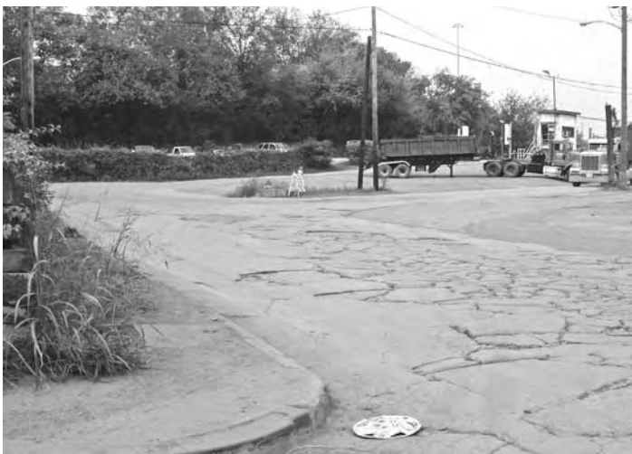
The condition of Richards Street, the only connection in the area, is another reason for the new road system.
