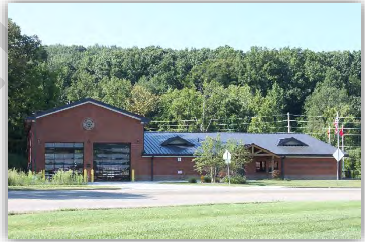
Image 4. The Karns Volunteer Fire Department Station 2 was constructed in 2013 to better serve the growing population in the Hardin Valley area.
