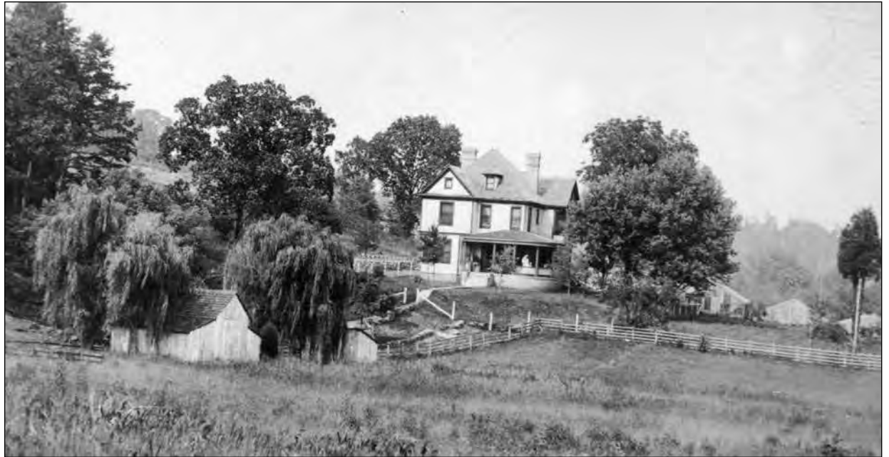
Vincent Babelay house and greenhouse (c. 1913), Washington Pike at Babelay Road, Ritta Community Courtesy of the Knox County Two Centuries Photograph Collection, McClung Historical Collection, Knox County Public Library System
