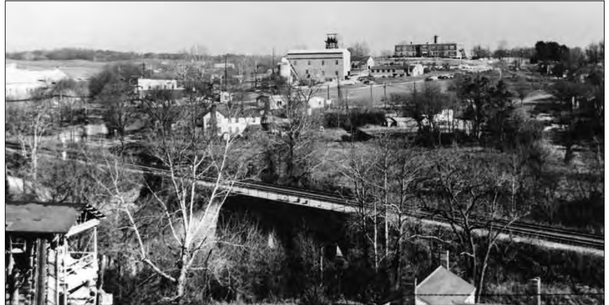
Mascot: Shows Southern Railroad tracks over Flat Creek, McMillan house (in center, with chimney), and McMillan Cemetery in right foreground in trees. Courtesy of the Knox County Two Centuries Photograph Collection, McClung Historical Collection, Knox County Public Library System
